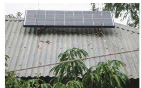
Bank financed renewal PV Solar Home System
